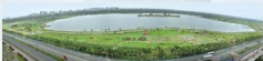
The project is located opposite to the Salt Lake VIT campus of Ecopark.
